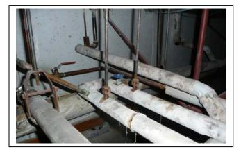
Photo 1. Mould growth on fabric jacketing due to high relative humidity in the crawlspace. As the relative humidity increased, the moisture content of the fabric increased to a level where mould spores on the fabric could germinate and colonize.
