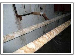
Photo 2. Staining on pipe insulation jacketing indicates condensate dripping from above. Note also the staining on the foundation wall insulation resulting from corrosion of the piping.
