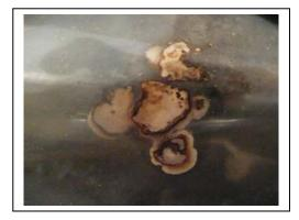
Photo 3. Fungi growing on a concrete footing beneath polyethylene ground cover material. The ground cover is resisting the ingress of moisture into the crawlspace as intended by the National Building Code of Canada. In the absence of moisture the fungal spores would not germinate and colonize.
